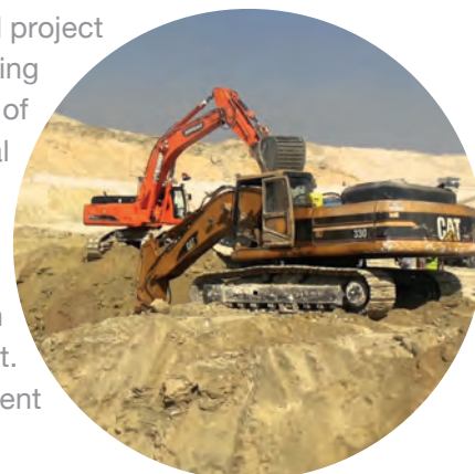
Dredging works at the new Suez Canal
