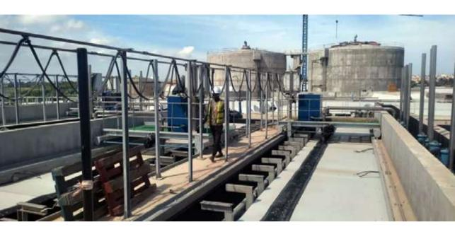
The only wastewater treatment plant in the northern system of the city of Dakar with a capacity of 19,200m3/day operated with a volume load equal to 208%. Hence a strong degradation of its purification performance and the depollution rate.
